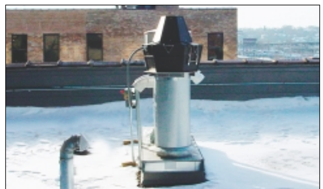
Above: Tjernlund's VSAD Auto-Draft Inducer terminates the stack connected to six boilers. It is controlled by a CPC-3 Constant Pressure Controller.
