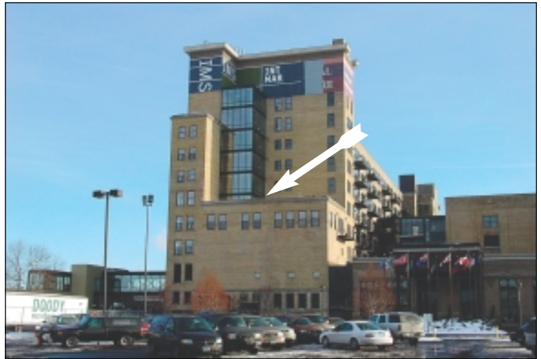
Arrow points to roof where wind swirled to create downdraft and boiler shutdowns prior to installing a mechanical draft system using Tjernlund's modulating draft inducer and CPC-3 Constant Pressure Controller.
