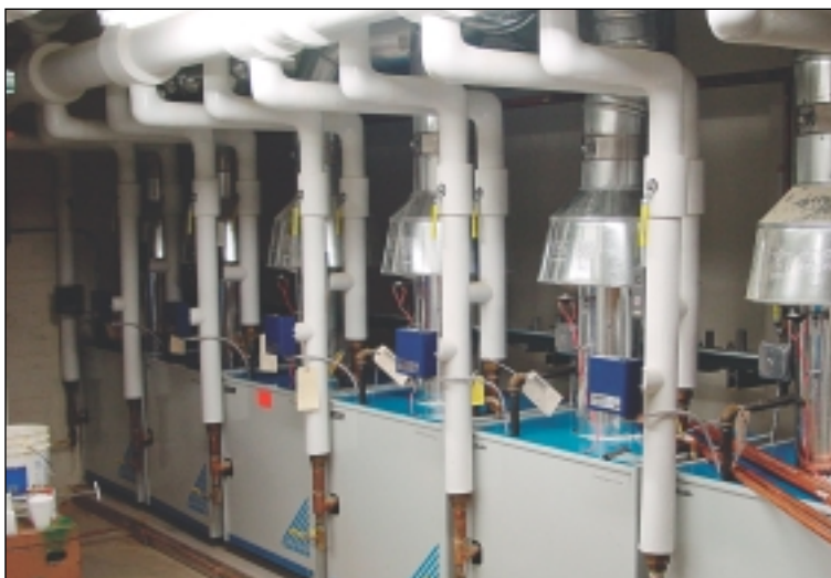
Above: Tjernlund's VSAD Auto-Draft Inducer terminates the stack connected to six boilers. It is controlled by a CPC-3 Constant Pressure Controller.
